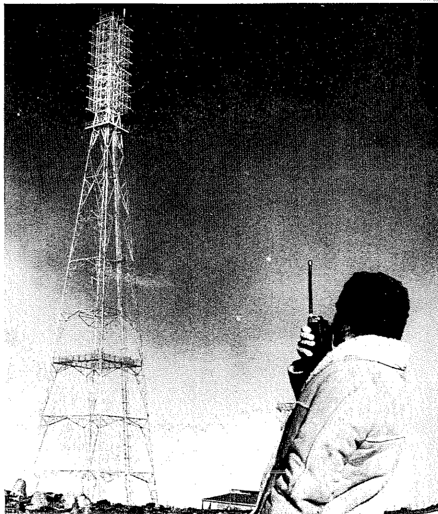
Inspecting the aerials of VK7RHT.
