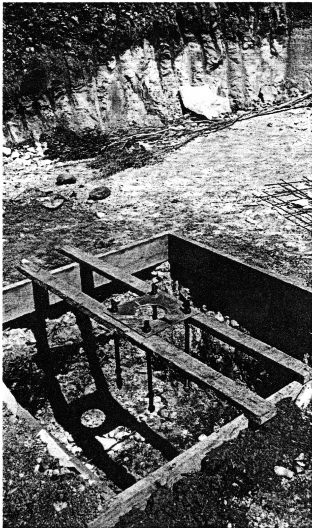
Mast thrust block formwork and steelwork in place, Strahan.
