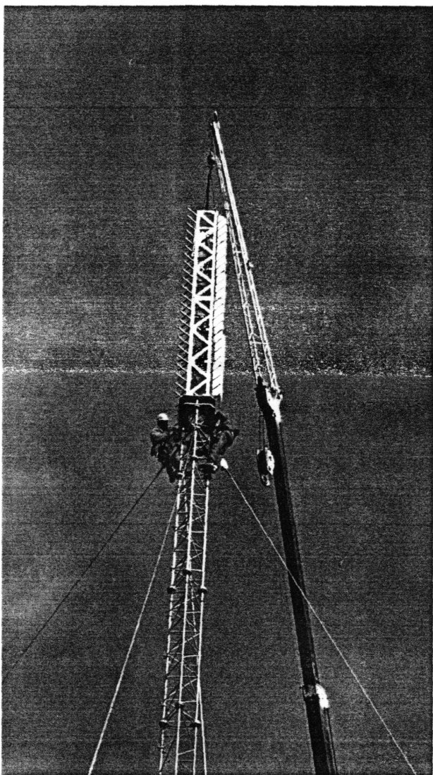
UHF antenna being placed in position on mast at Taroona.
