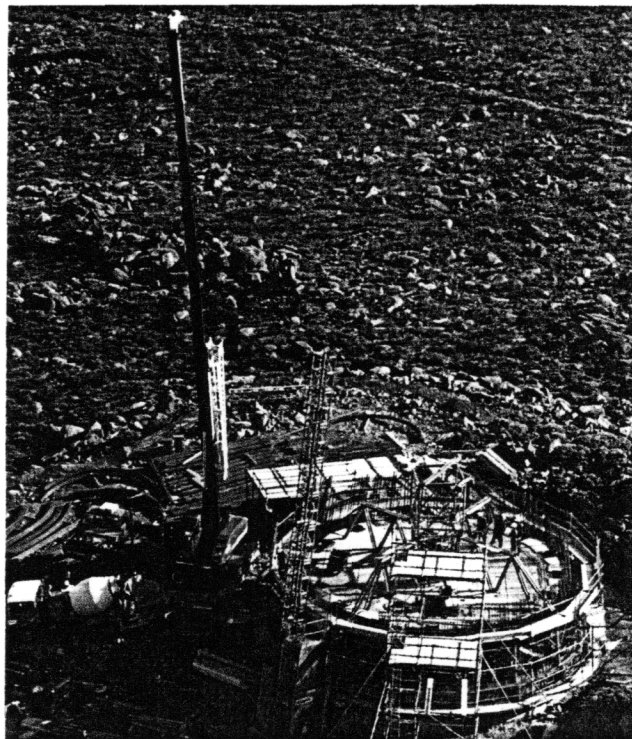
Final stage of slipform assembly and adjustment.
