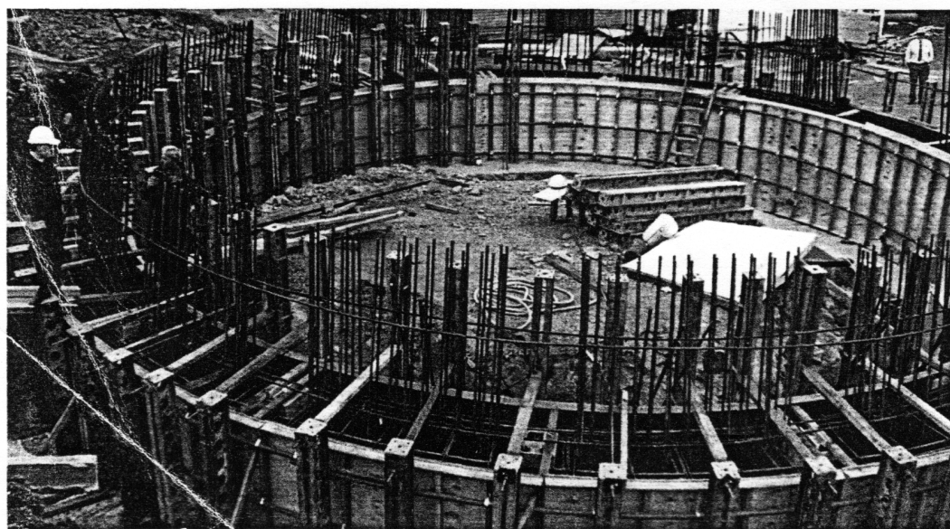
Formwork and reinforcement set up prior to pouring foundation ring beam.
