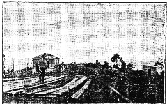
Preparing for the construction of the two 140-foot masts which will carry the aerial system. The aerial will be of the "T" type.
