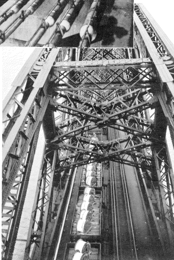
Fig. 4—Forth Bridge — Laying cables from trucks (view taken from top of south pier).
