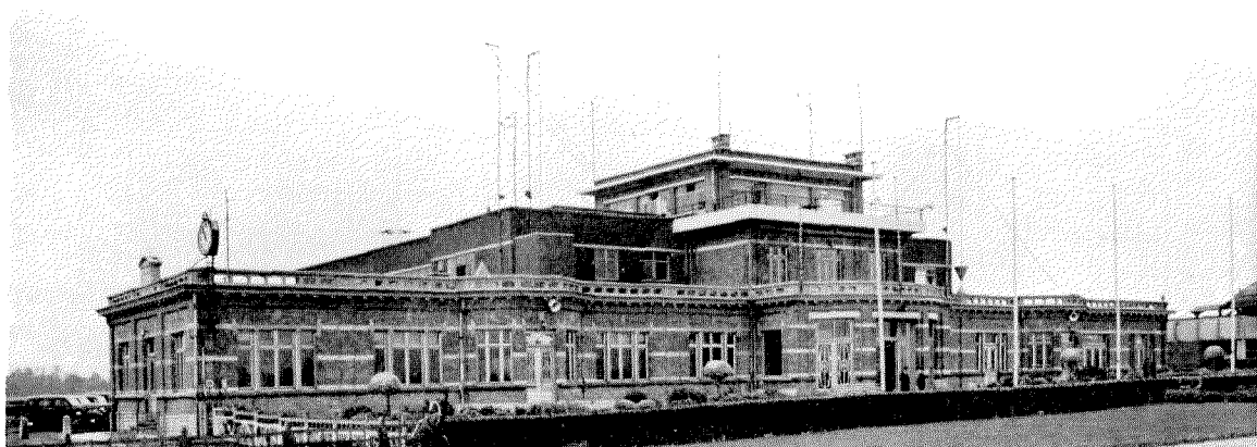
Administration Building—Belgian Air Ministry, Brussels.
